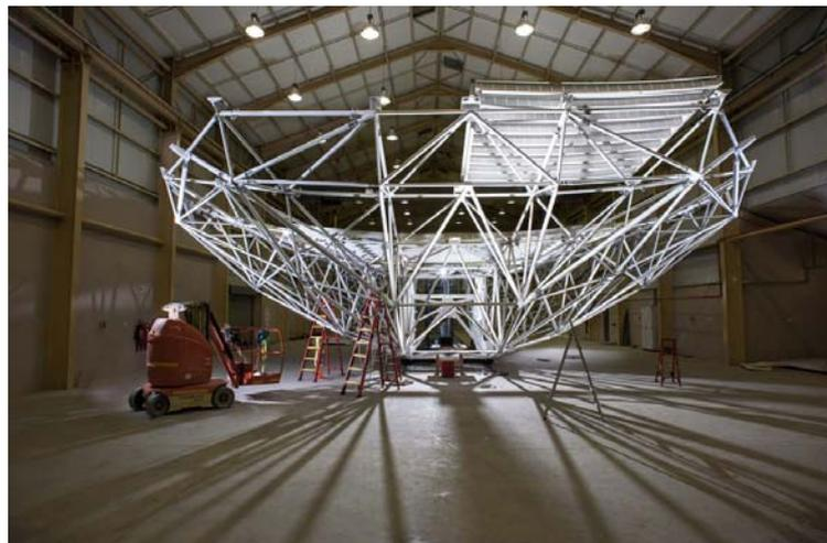
*The dishes are carefully assembled onsite. The margin of error allowed while constructing them is very small, as the functioning of the dishes depends on precision of movement and stability. (Photo courtesy of SKA South Africa)*
